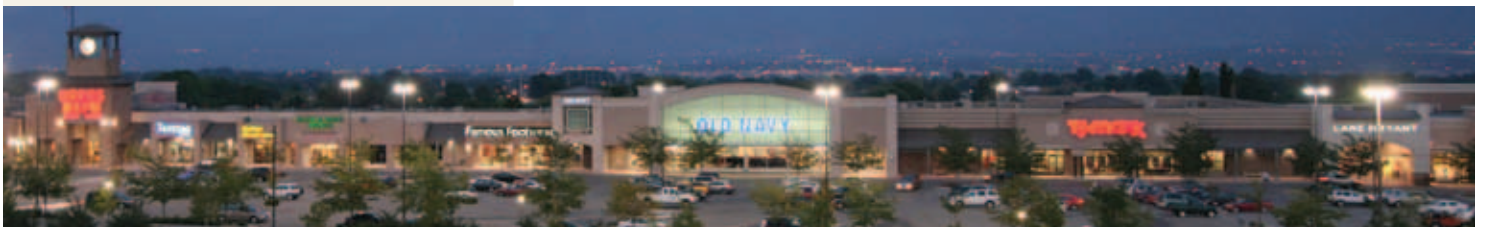
Jordan Landing, the state's largest commercial power center, features 1.4 million square feet of shopping and an additional 1.5 million square feet of office space.
